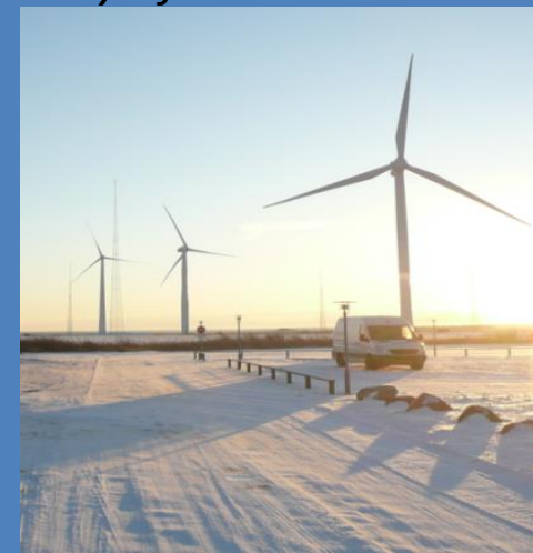
On-site tests on renewable sources
