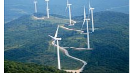
Large-scale Onshore Wind Power Project
