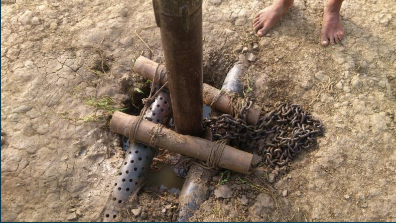
Pipe boring process
