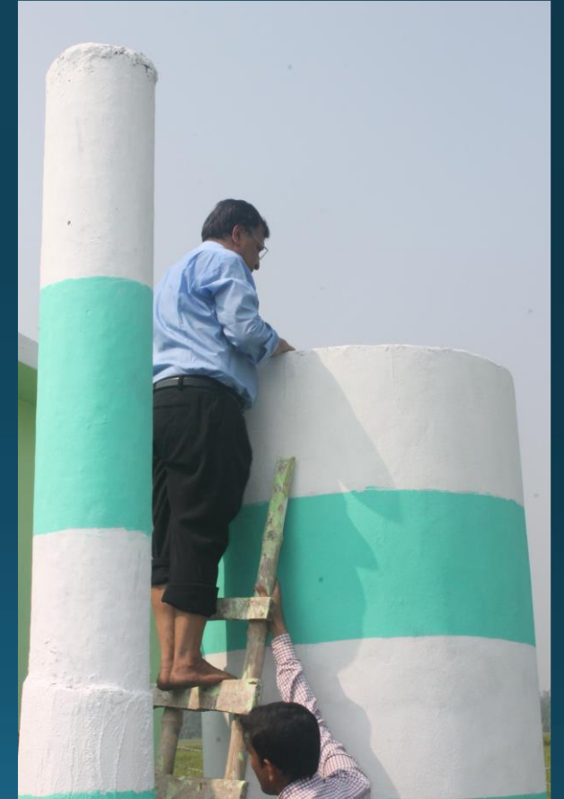
Inspecting water reserver tank
